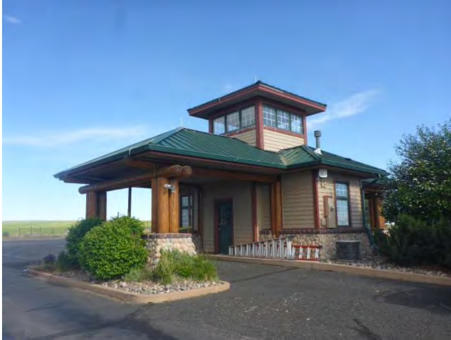
Figure 1. Overview of entrance building (looking northwest)
