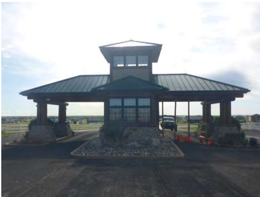
Figure 2. Overview of entrance building (looking east)
